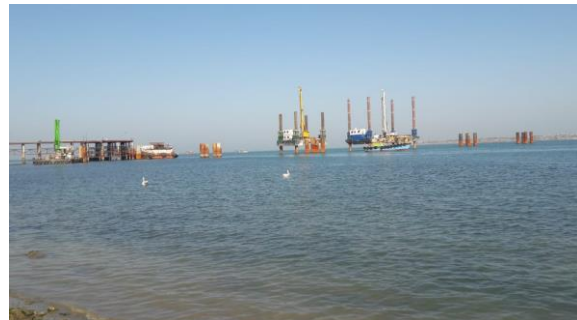
Figure 5.14 hall site view
