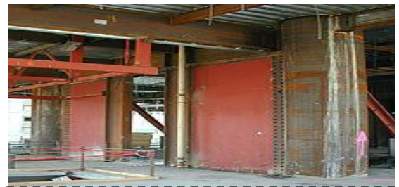
Fig.14.5 Infill Shear Trusses
