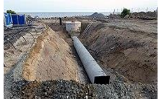
Fig14.9 Sewers Under Construction Water Table
