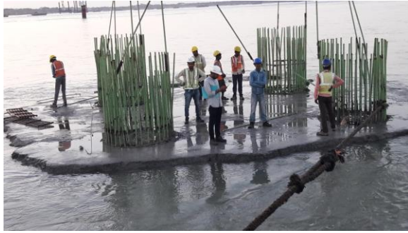
Figure 5.11 pile caste
